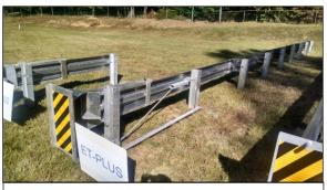
**Figure 9:** Oblique view of an exemplar 10 cm (4 in) ET-Plus installation.
