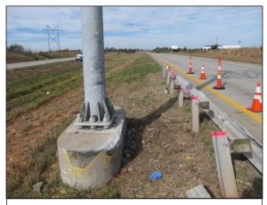
**Figure 7:** Northwest-facing view of the impact damage and physical evidence on the concrete base and pole.
