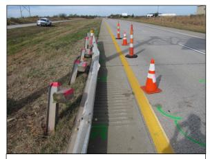
**Figure 8:** Northwest-facing view of the deformed guardrail at Posts 21-25.
