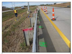
**Figure 11:** Northwest-facing image along the deformed guardrail from Post 13.
