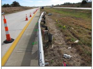
**Figure 10:** Southeast-facing image along the deformed guardrail from Post 13.
