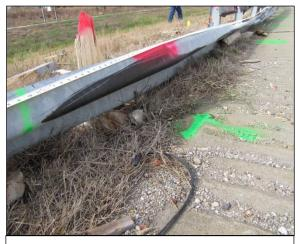
**Figure 5:** Northwest-facing view of the W-beam in the vicinity of Post 7 and the black transfer of the Chevrolet's right front tire.
