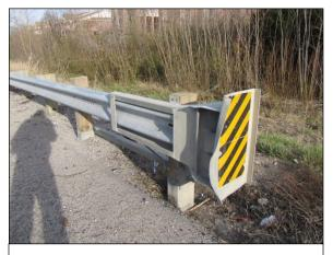
**Figure 4:** Image depicting an exemplar ET-Plus installation located near the crash site.
