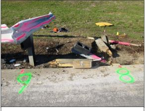
**Figure 10:** View of deformed Post 8 and Post 9 at the time of the SCI crash site inspection.
