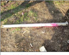
Figure 9: Displaced ground angle strut.
