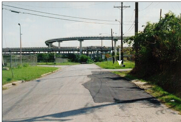
Figure 1: Case vehicle's southward travel path in southbound lane; Note: arrow indicates location of impact with culvert (case photo #01)
