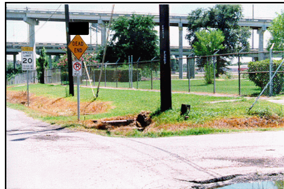
Figure 2: South-southwest view from southbound lane showing case vehicle's path of travel to impact with culvert on southwest corner of "Tee" intersection; Note: front right tire track in mud (case photo #03)
