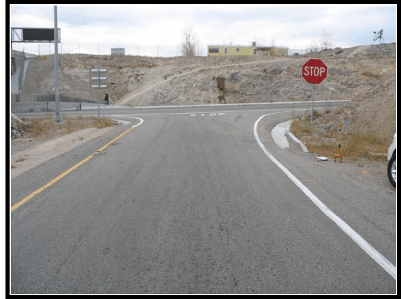
Figure 2. Westbound approach to end of exit ramp
