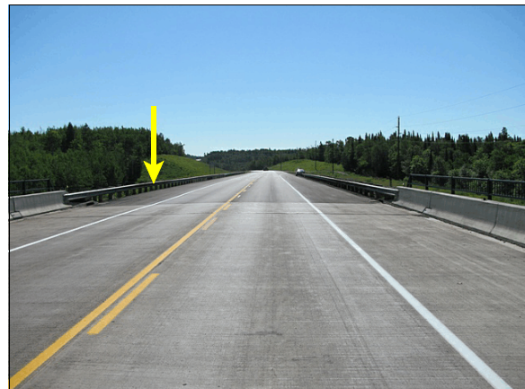
Figure 2: Approach of the ambulance eastbound on the bridge; arrow shows the area of the crash
