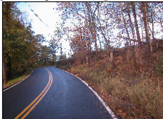
Figure 3. Right side road departure.
