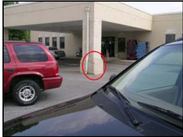
Figure 3: View of the POI (highlighted).
