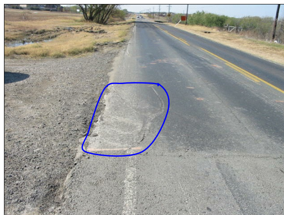
Figure 4: Impact evidence (circle) on south edge of pavement from Mack truck's left rear as a result of truck's rollover in eastbound lane; Note: POI mark indicates cab's impact area (case photo #14)
