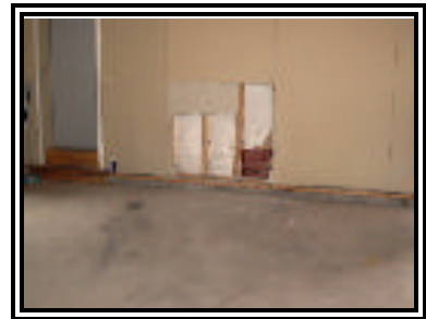
Figure 3. Impact damage to the garage wall.
