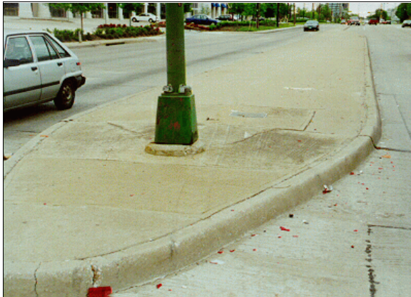
Figure 10: Case vehicle's path of travel into median after initial and side slap impacts with other vehicle; Note: case vehicle impacted the curb and then sideswiped the utility pole
