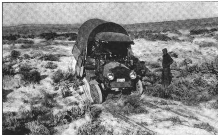
SHOWING HOW THE TRUCK WAS RACKED AND TWISTED
