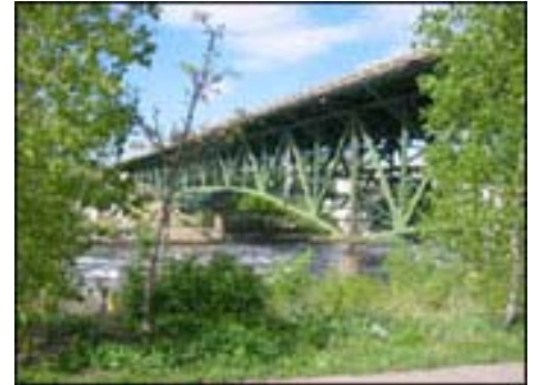
Rebuilding the I-35W bridge over the Mississippi River in Minneapolis will be the first project developed under the new Design-Build Rules
