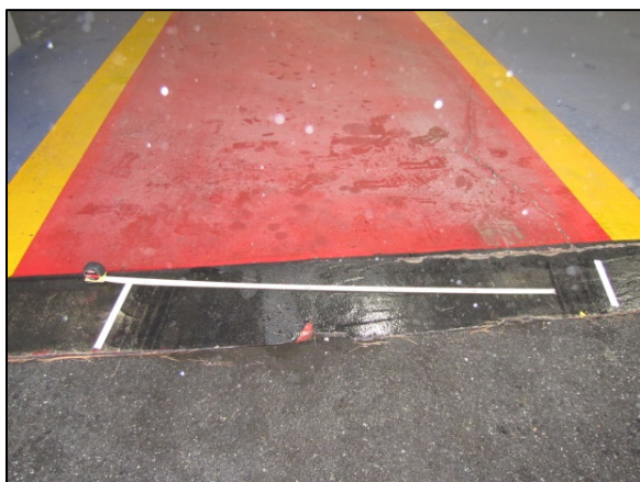
Figure 8: North-facing image of the tire marks at the entrance to Lane #6. Note the angled orientation of the marks relative to the travel lane.
