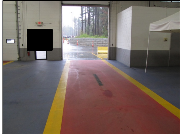
Figure 4: South-facing lookback view from the center of the building along the Jeep's path at Lane #6.
