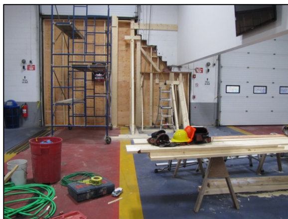
Figure 9: North-facing image of the fractured exit wall at the point of impact (under repair at the time of the SCI inspection).
