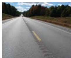
2-Lane Roads 80–90km/h (Milled rumble strips)
