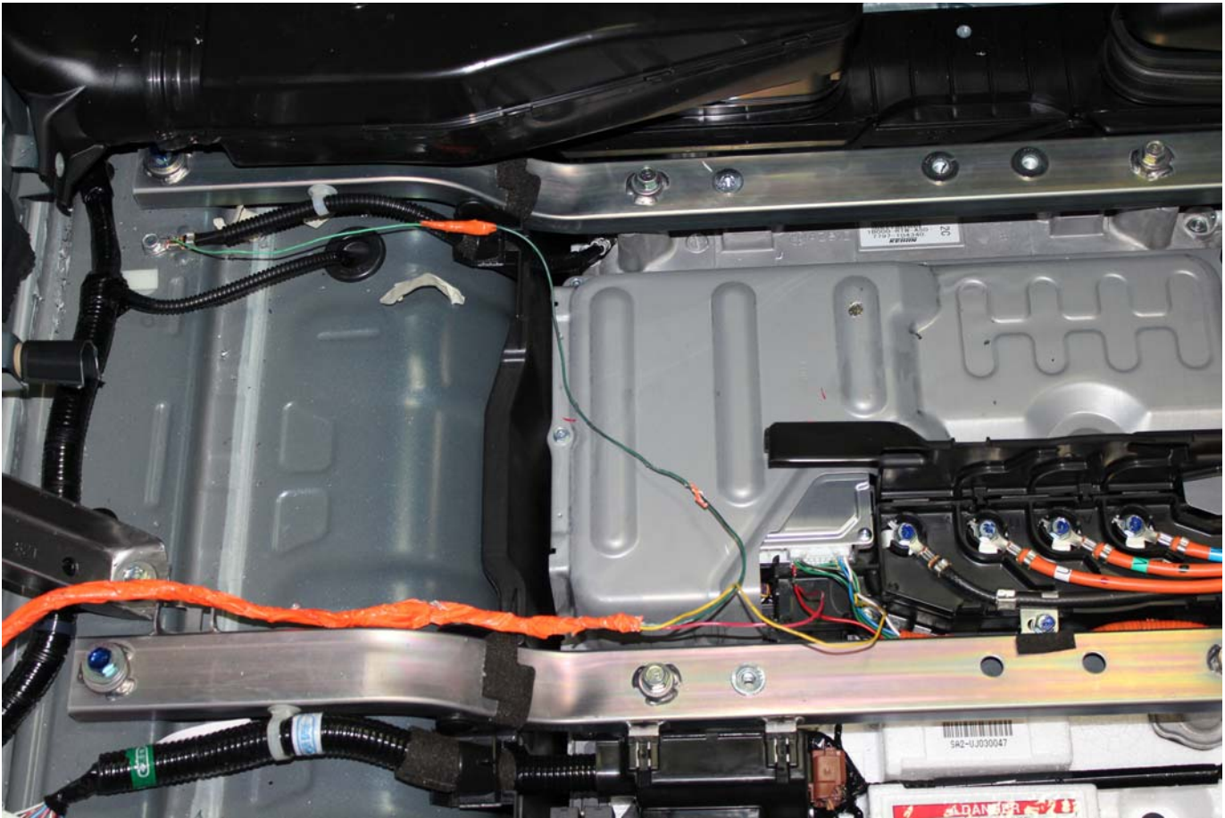
Ground Location/Close-up of Leads Attached
