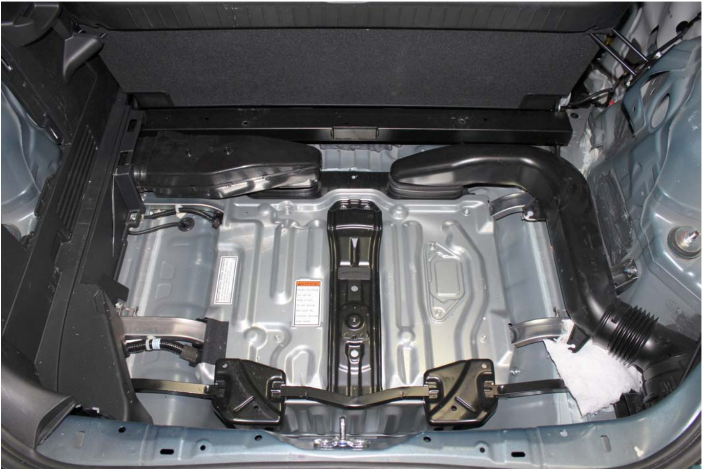
Post-Test View of Propulsion Battery
