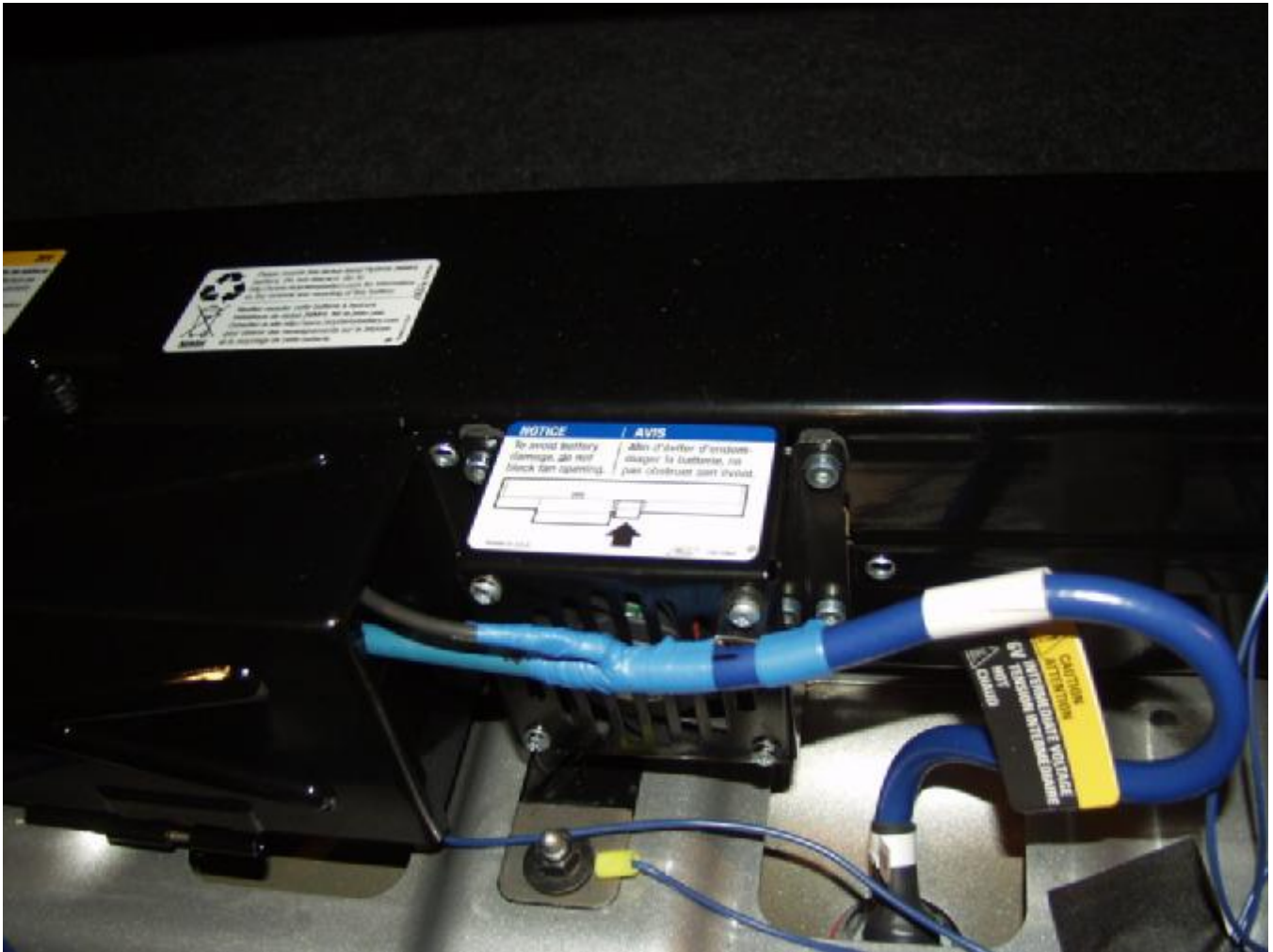
Figure A-37: Pre-Test High Voltage Interconnect View
