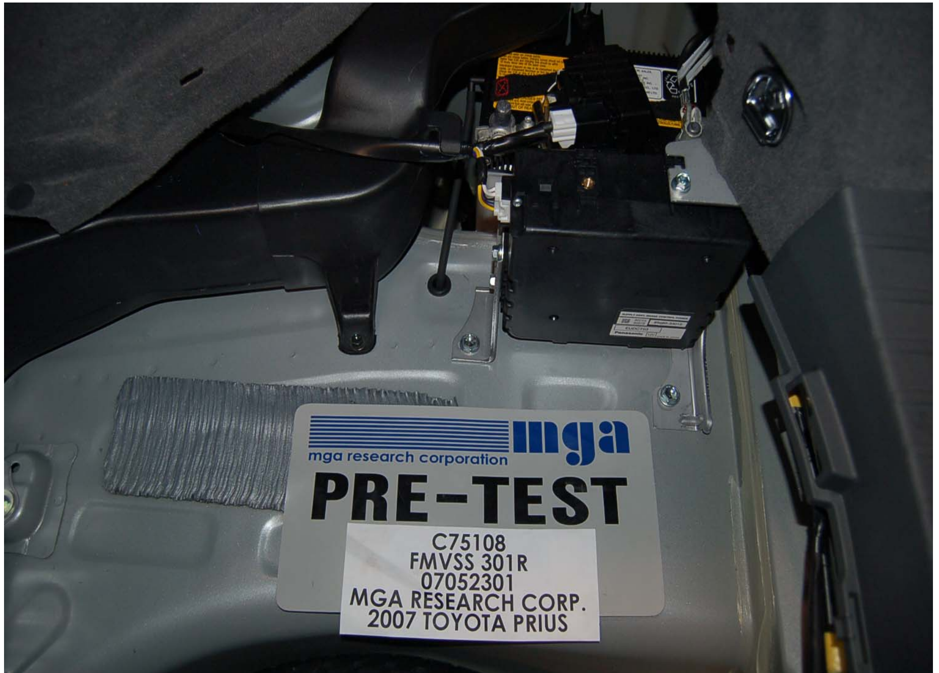
Pre-Test Propulsion Battery Venting System
