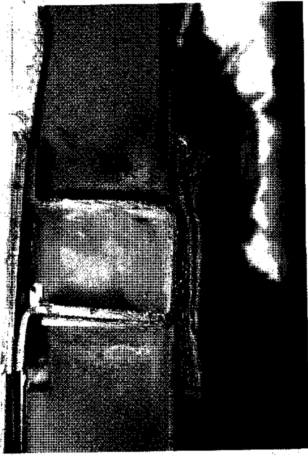
End View of Joint #1
