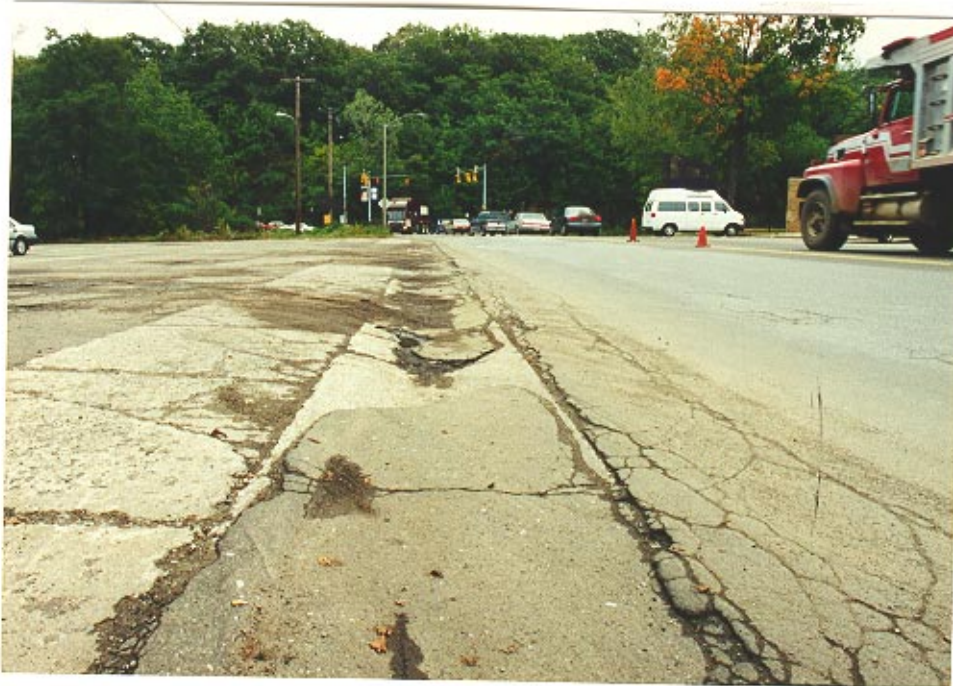
4. Longitudinal view of the concrete rain gutter in the area of the left turn maneuver.
