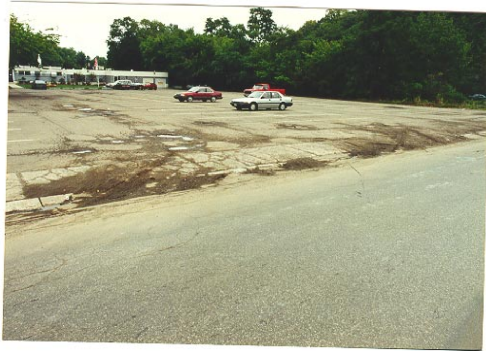
3. Left turn maneuver into the parking lot.
