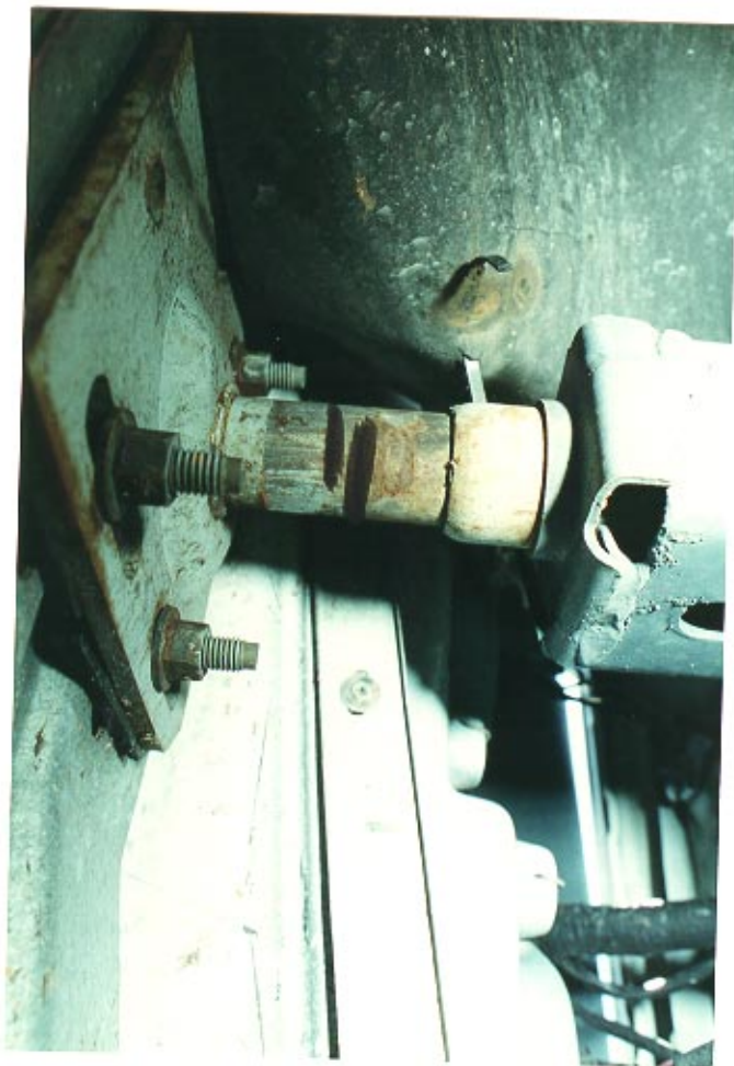
15. Compression of the left front bumper energy absorbing device.
