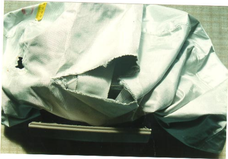
31. Close-up view of the membrane tear.
