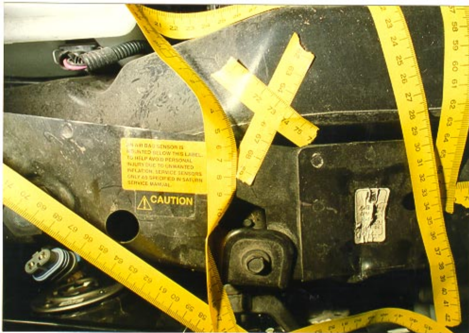
34. Close-up view of air bag discriminating sensor and radiator support damage.
