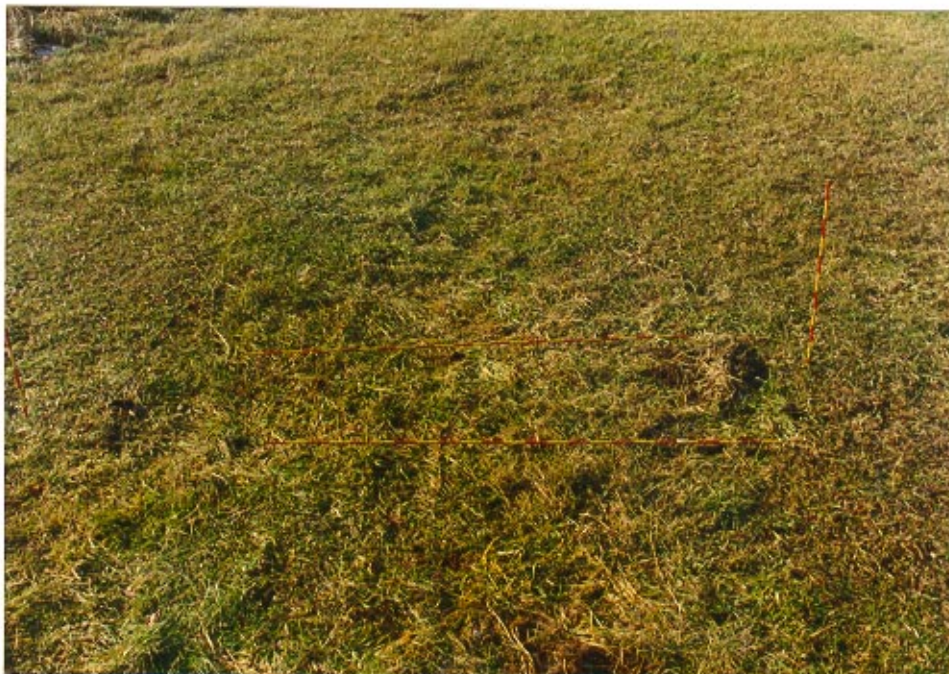
14. Close-up view of pedestrian's FRP.
