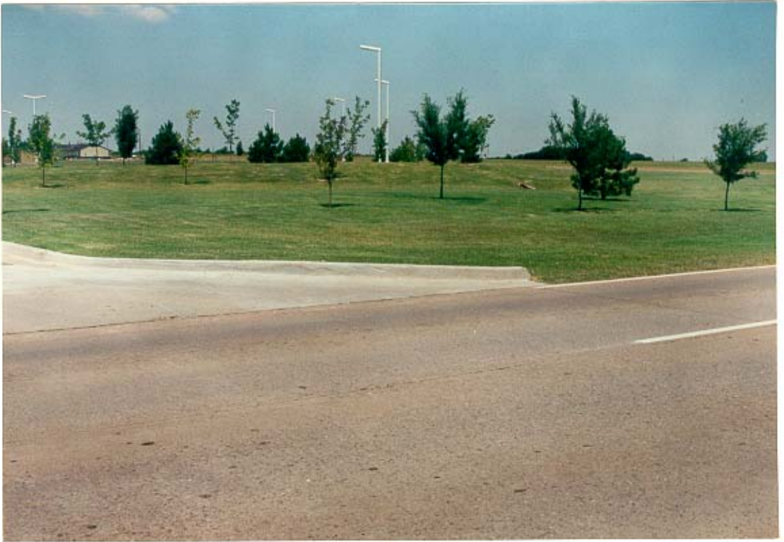
View to northwest approach to curb
