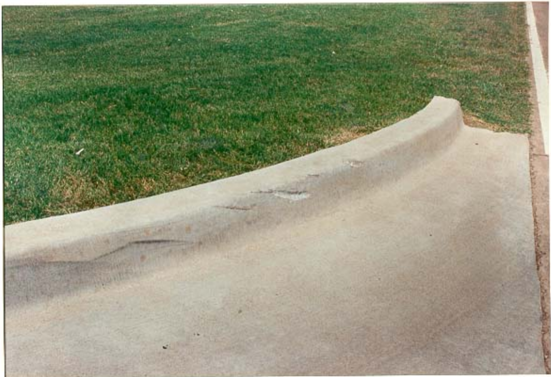
Closeup of contact with curb
