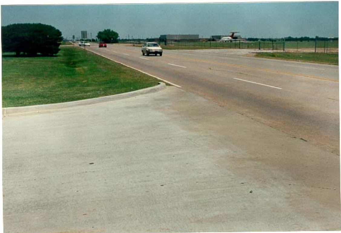
Lookback from area of final rest to north
