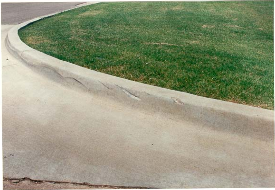
Closeup of contact with curb
