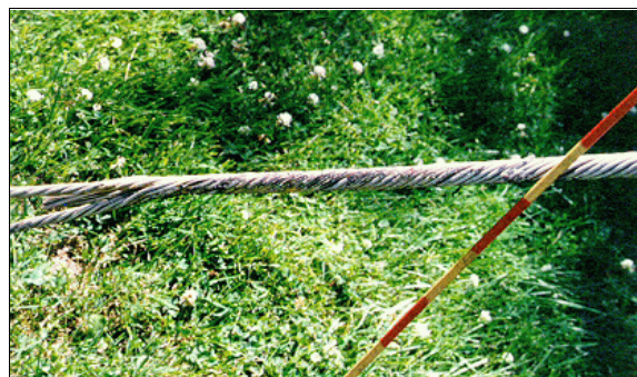
Figure 7: Close-up of guy wire section damaged by impact with case vehicle (case photo #07)
