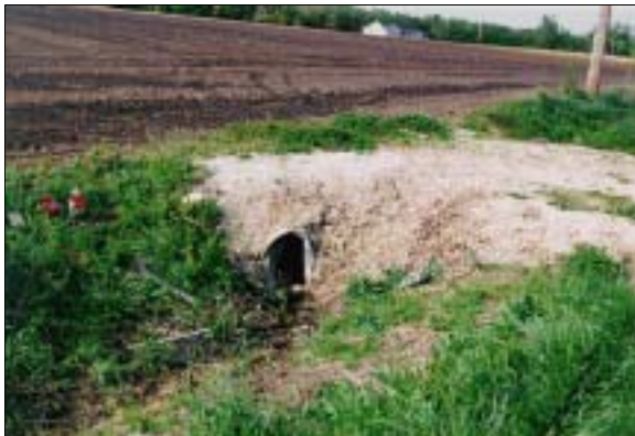
Figure 6: Culvert's embankment on north roadside that was impacted by case vehicle; Note: case vehicle came to rest on other (east) side of gravel drive (case photo #05)
