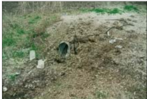
Figure 7: Coroner's photo, looking northeastward, showing culvert/embankment impacted by case vehicle; Note: disruption of embankment that occurred during crash (case photo #48)
