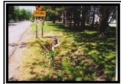
Figure 2. Impacted concrete culvert.
