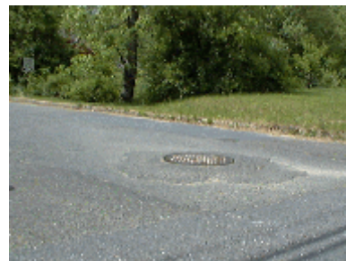
Figure 6. Raised manhole in the left turn path of the Plymouth Neon.
