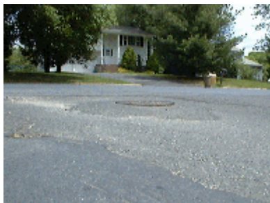
Figure 5. Look back view of the raised manhole and pavement edge.
