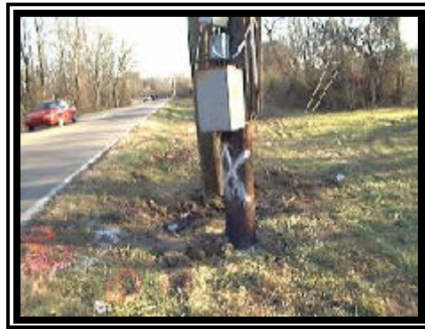
Figure 2. Struck utility pole.
