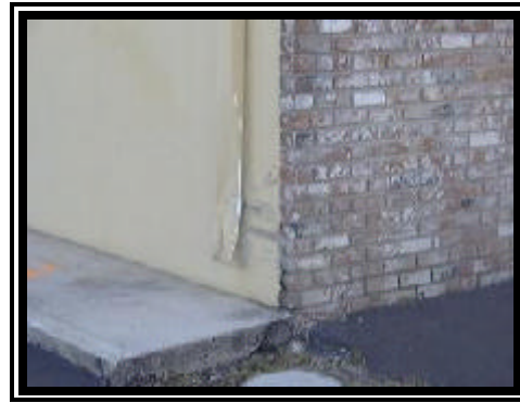
Figure 3. Struck building (impact #3).
