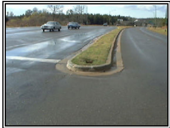
Figure 2: View of the barrier curb and the area of the Pontiac's final rest.
