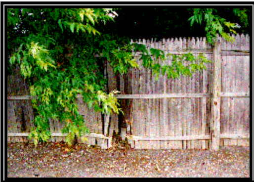
Figure 2: Close-up view of the fence at the point of impact taken during the police investigation.
