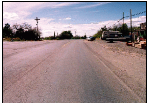
Figure 1. Roadway and impact area.
