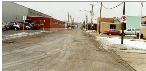
Figure 1: Case vehicle's southward approach path; Note: case vehicle struck Chevrolet which was illegally parked along east (left) side of roadway and then struck and came to rest near corner of red brick building in background (case photo #01)
