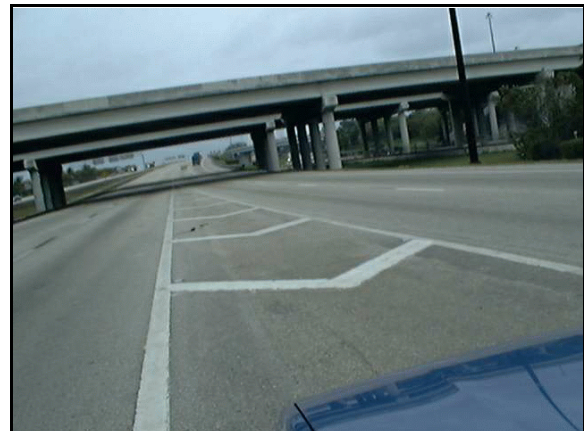
Figure 1: Case vehicle’s westbound approach toward impact with bridge pillar on right
