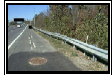
Figure 1. Guardrail impact area.
