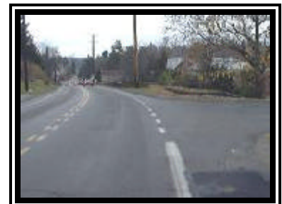
Figure 1. Northbound approach for the 1998 Buick LeSabre (impacted pole in background).
