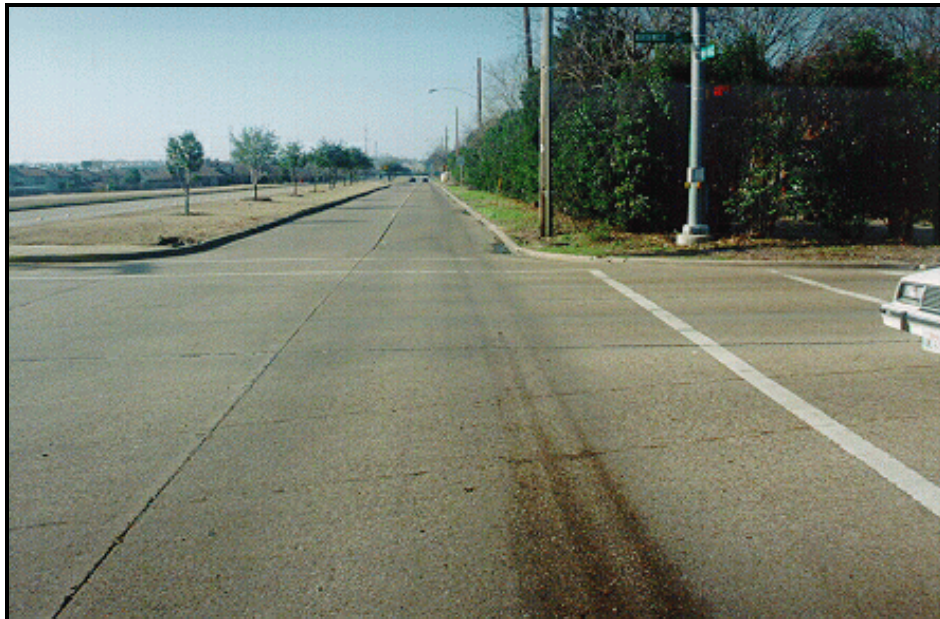
Figure 1: Vehicle #2's west-bound approach with point of impact for first harmful event at middle foreground (case photo #5)
