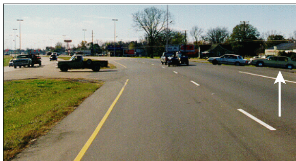
Figure 1: Case vehicle's southbound travel path in inside lane of left-hand curve; Note: roadway's +8% superelevation and the 8% positive grade on the west leg (arrow) as Chevrolet attempted to cross the roadway from right-to-left, heading eastward (case photo #01)
