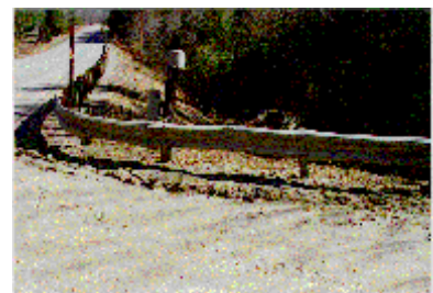
Figure 4. Struck guardrail.
