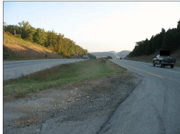
Figure 2: View south in the area where the Toyota departed the roadway
