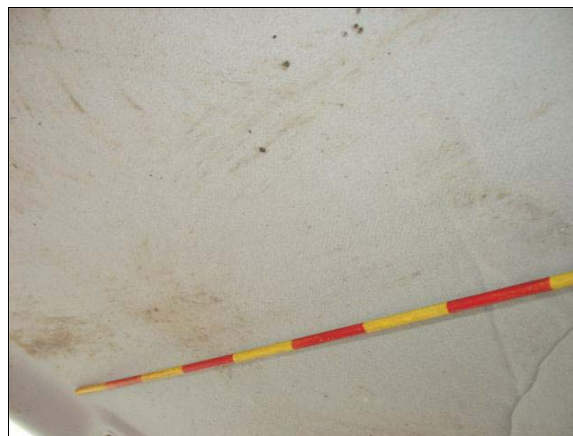
Figure 7: Roof contact above driver area
