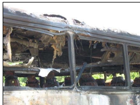
Figure 7. Burn-through of the right aluminum roof panels.
