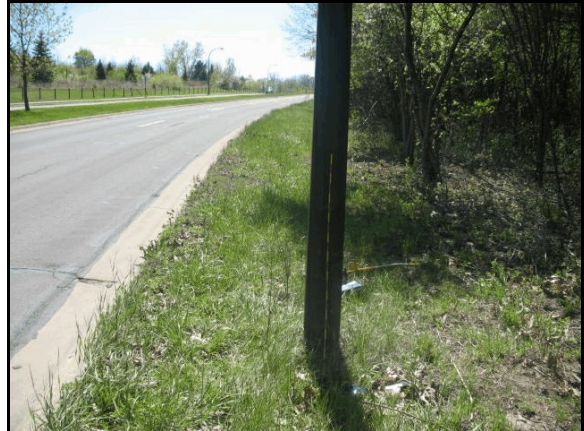
Figure 3: Steel luminaire support pole; hexagonal cross-section, approx. 18 cm (7 inches) diameter
