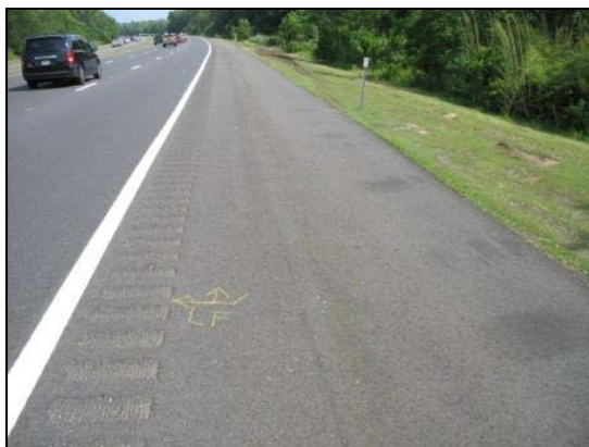
Figure 6: Departure of the motorcoach onto the west shoulder.
