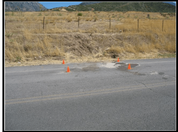
Figure 4. Final rest and impacted barbed wire fence (looking east)
