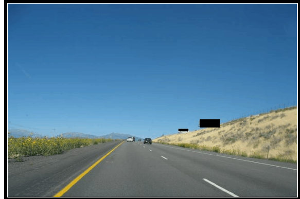
Figure 2. Northbound approach to left side roadway departure
