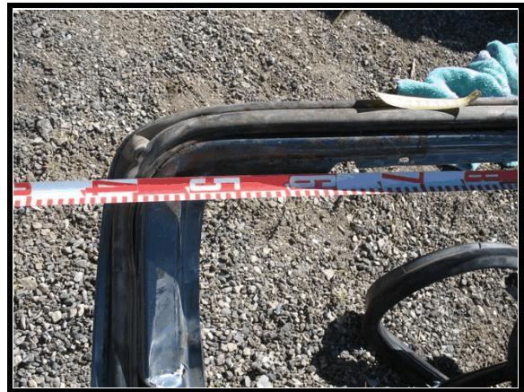
Figure 17. Contact to left upper window frame
