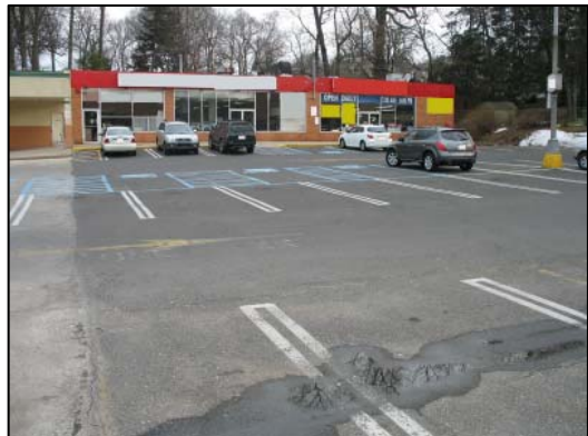
Figure 4: View looking eastward across the southern half of the parking lot.
