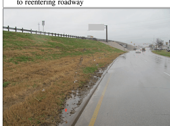
Figure 5: Lexus departs left (north) side of roadway and approaches impacts
