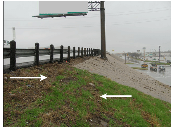
Figure 7: Approach to impact with guardrail posts, arrow on left shows left side tire track; arrow on right shows right side tire track
