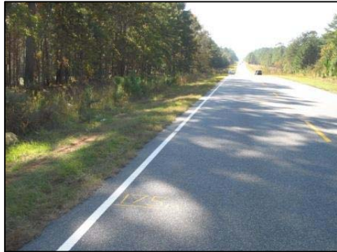
Figure 2. Overall westbound view of the crash site.
