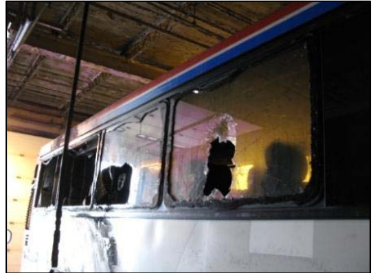
Figure 6. Firefighter induced damage to the right side glazing panels.
