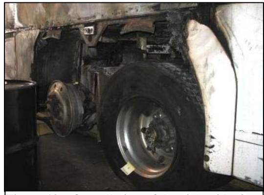
Figure 10. Overall view of the right side tire and tag axle wheel damage.
