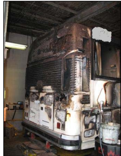
Figure 3. Fire damage to the back of the MCI motorcoach.
