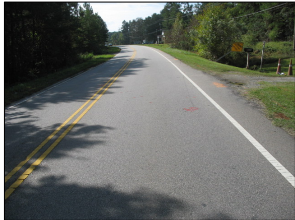
Figure 2: Southbound trajectory view of the crash site.
