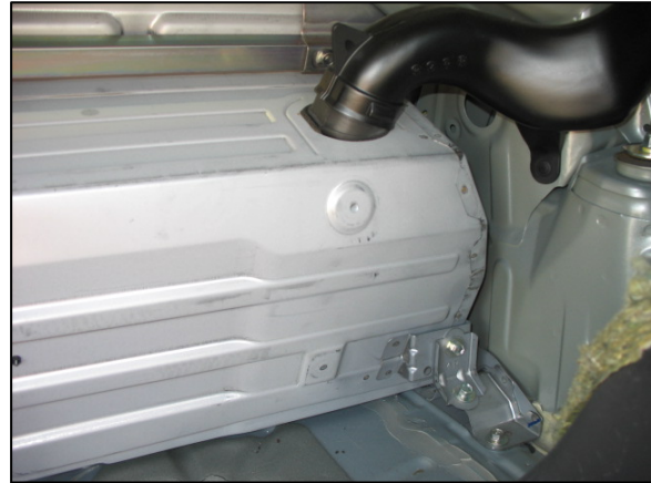
Figure 7: Right half of the hybrid battery pack and the ventilation exhaust.
