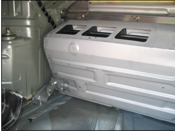
Figure 6: Left side of the hybrid battery pack and ventilation intake with the duct removed.
