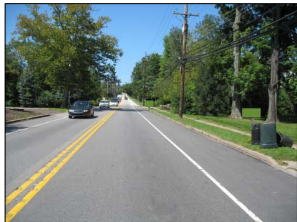
Figure 2: Westbound view at the crash site.
